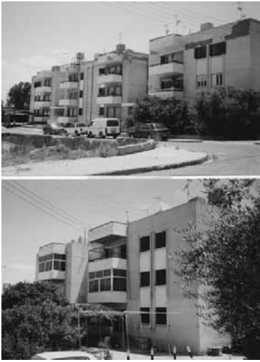
Figure 3. A typical three storey building in refugee estate and typical interventions by the residents to gain some space.
