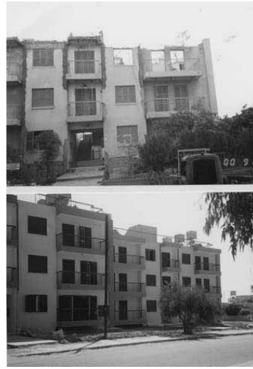
Figure 4. A typical three storey building in refugee estate and typical interventions by the residents to gain some space.
